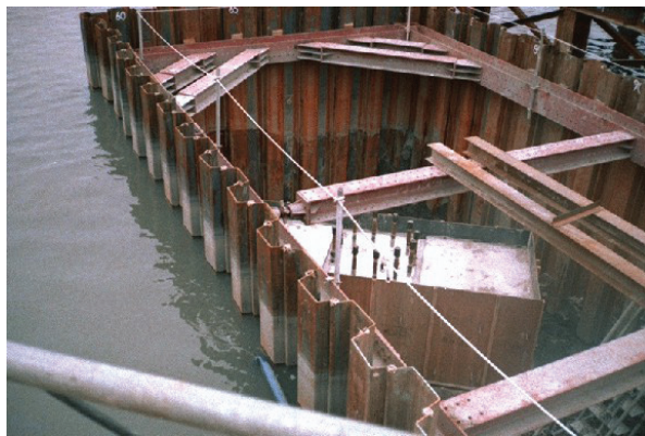
Sheet Pile Interlock
