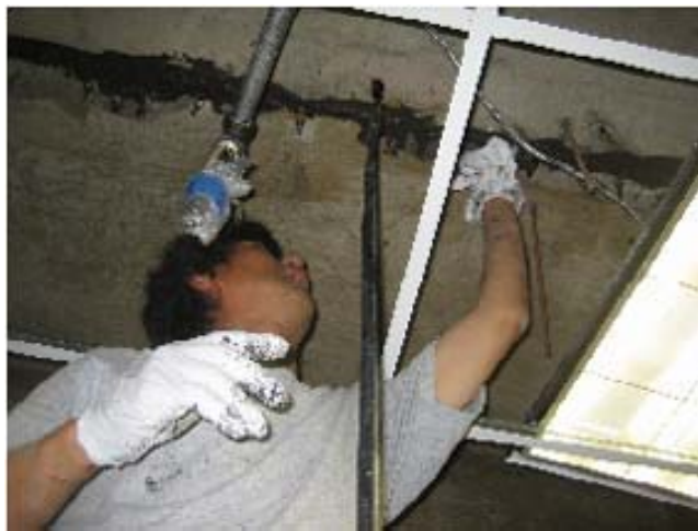
Horizontal Ceiling Injection with high pressure injection pump
