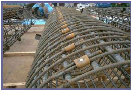
Rebar-Cage for Cast-in-place concrete pile
