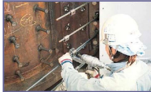
Reinforcements for SRC beam-Column joint
