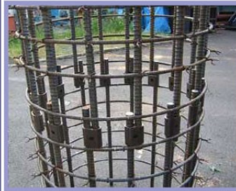
Rebar-Cage for Cast-in-place concrete pile
