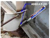
Use to fill in rough areas when using Adeka strip products. Apply on PVC waterstop weld seams.
