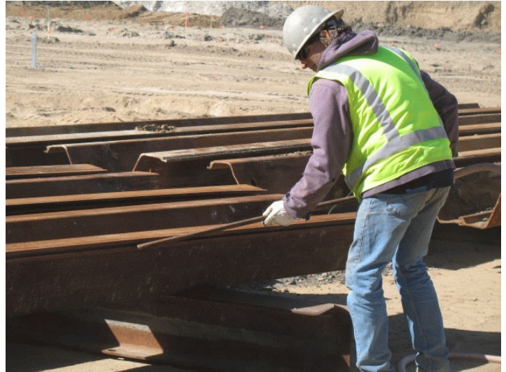
Remove any loose debris by compressed air.
