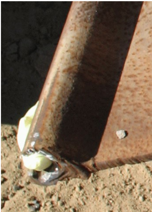
Plug ends with urethane foam in spray can, backer rod or bead of chalk
