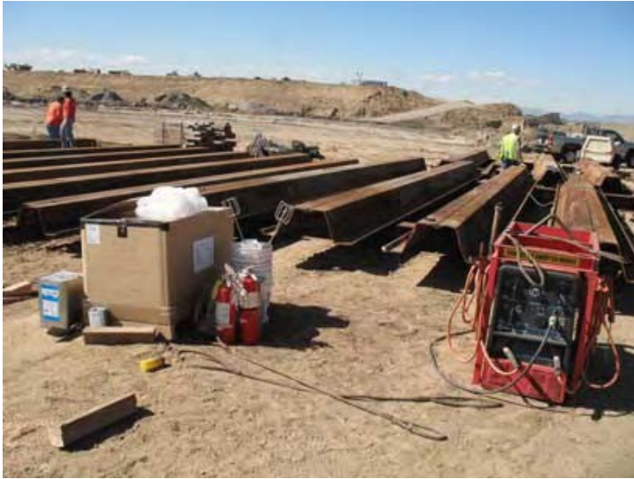
Place piles on parallel level H-beams.
