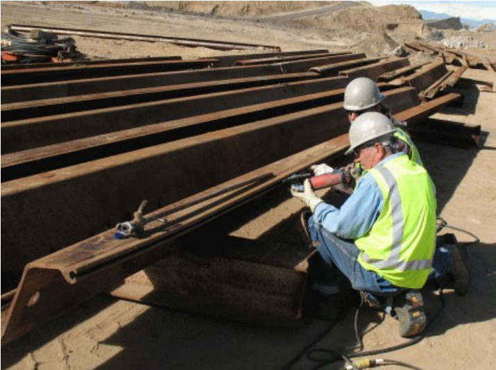
Cleaning socket with wire brush. IMPORTANT —Socket must be clean, dry, free from oils and any loose rust or debris.
